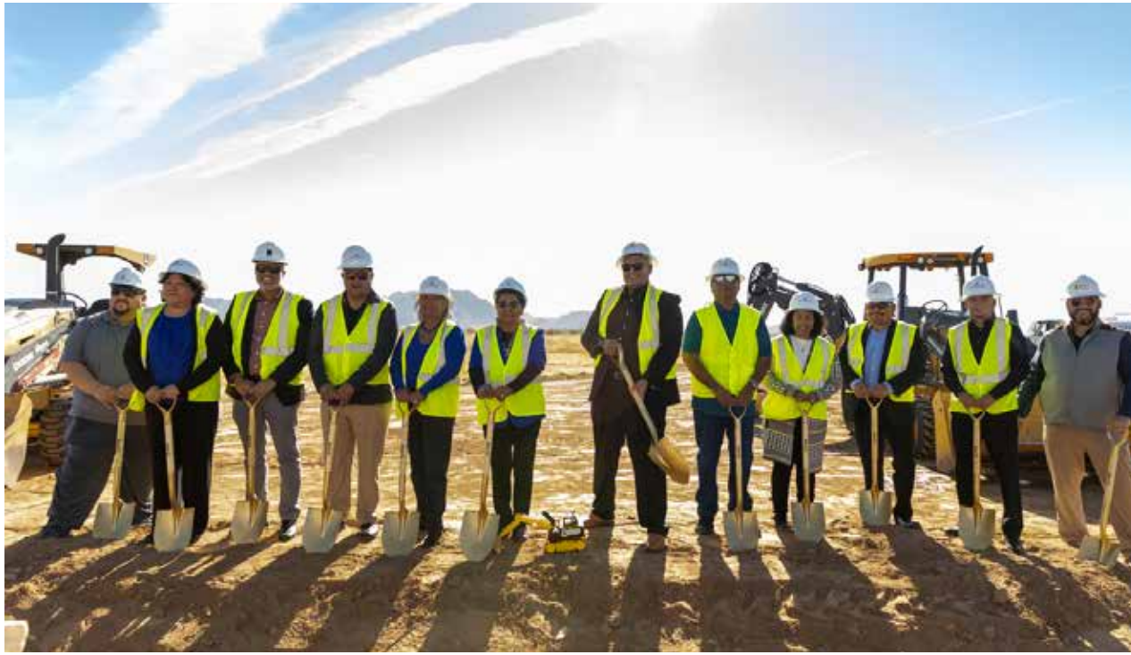
Tribal dignitaries and construction partners break the ground for the Sacaton Market on Dec 5, 2023, located on the southeast corner of S. Ocotillo Dr. and Bluebird Rd in District 3. Velia Moncada/GRIN
