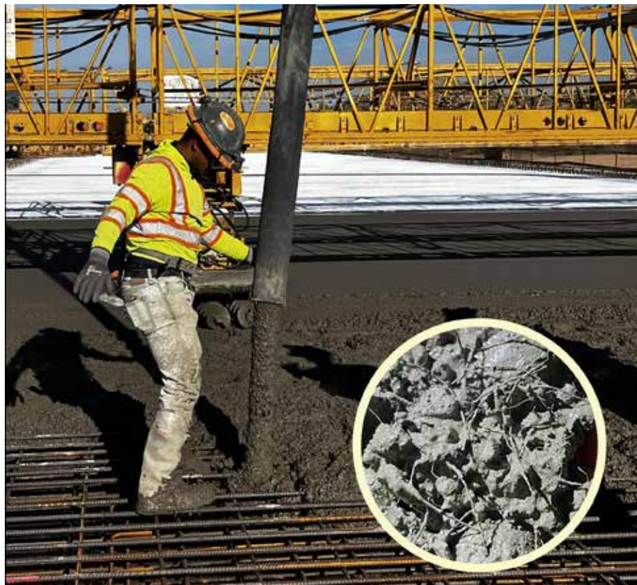
Crews placing concrete for the new bridge deck for the westbound I-10 Bridge Over the Gila River are adding something new. ADOT is using synthetic fibers in the concrete mix. These structural fibers help to reinforce the bridge deck, and increase resiliency against weather and traffic. The goal? Construct a longer-lasting bridge structure for Arizona motorists. The use of fiberglass in structural and pavement concrete is a technology that has been around for over 25 years. Photos Submitted by: ADOT
