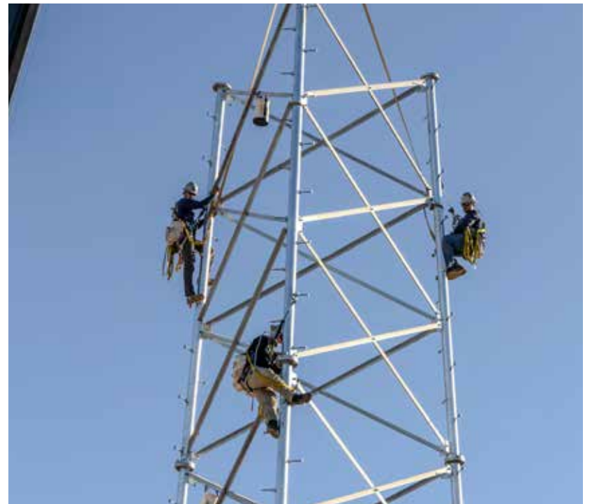
High above the ground, workers secure the antenna at 100 feet, with safety harnesses. Jeston Morris/GRIN
