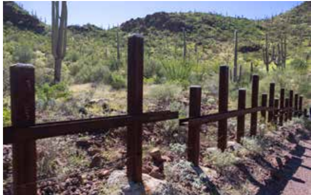
Barricades along the border on the west end of the Tohono O’odham Nation. Emma Hughes/GRIN
