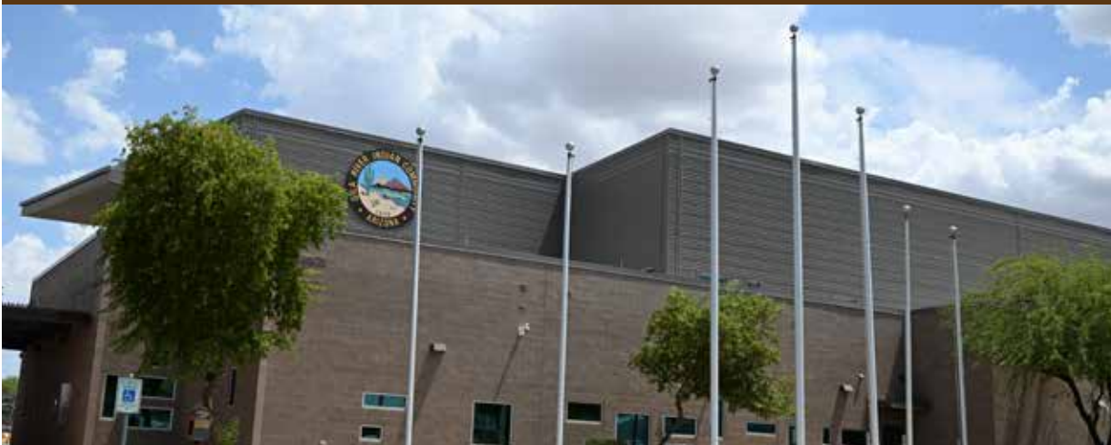
District 7 Service Center 8201 W. Baseline Road
